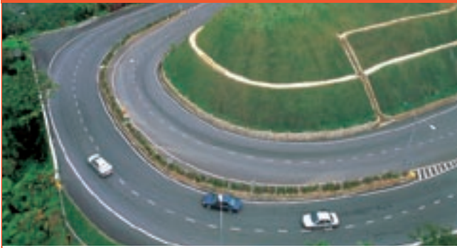
The completed dual carriage highway.
